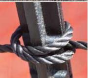
A clove-hitch at every post secures the non-conductive line in place.
